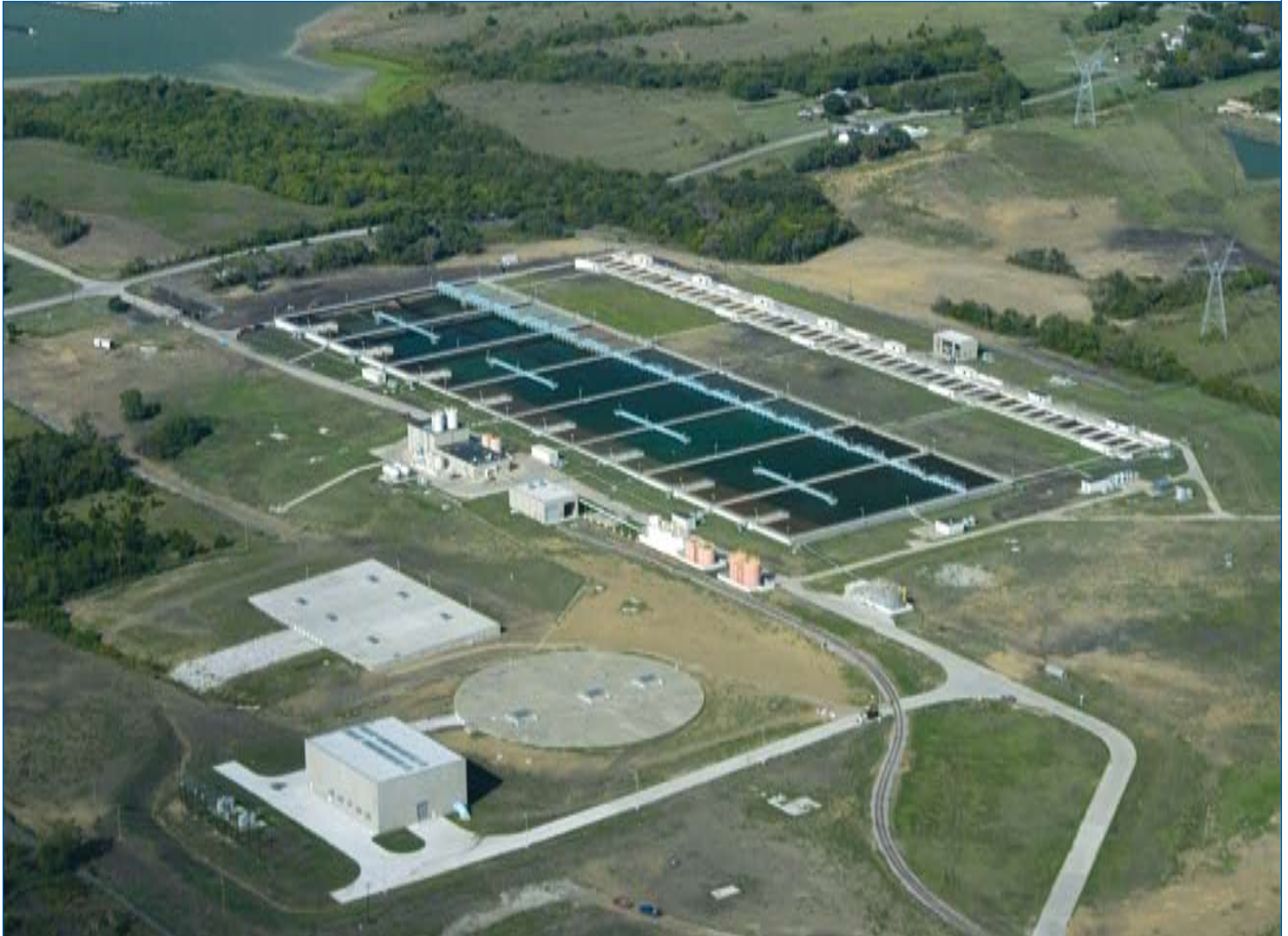
NTMWD's Water Treatment Plant III, one of three treatment facilities at the site in Wylie, treats up to 280 million gallons per day of a treated water supply of the total 630 MGD delivered to the region served
