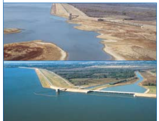
Jim Chapman Lake declined to elevation of 422.55' msl in October 2006 during drought conditions (top photo) as compared to full conservation pool elevation of 440' msl (bottom photo)
