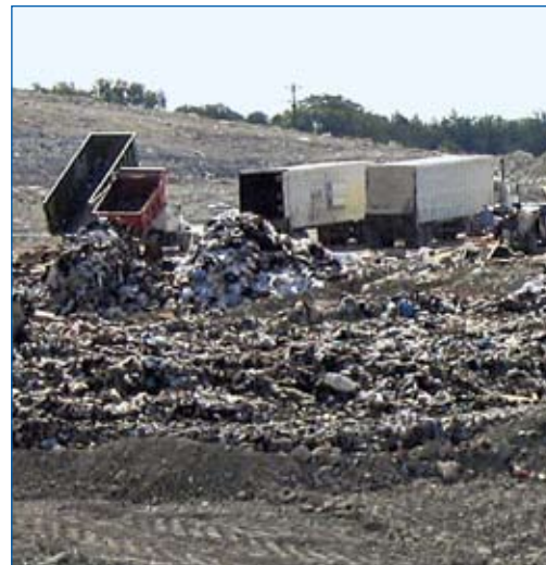
The 121 Regional Disposal Facility is expected to meet the solid waste needs of the area served by NTMWD for the next 40 years
