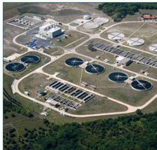
NTMWD's Wilson Creek Regional Wastewater Treatment Plant provides wastewater treatment under the strictest permit criteria in the State
