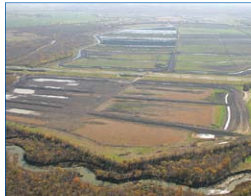
East Fork Raw Water Supply Project will utilize the environment through constructed wetlands to polish raw water supplies
