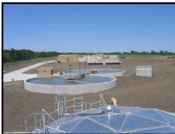
NTMWD's Muddy Creek Regional WWTP provides additional treatment for the Cities of Murphy and Wylie
