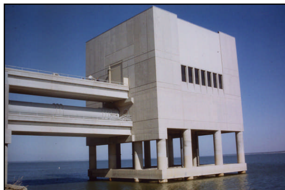
NTMWD's Raw Water Pump Station at Lake Texoma transfers raw water supplies to the Lavon Lake watershed. Raw water supplies flow down Sister Grove Creek into Lavon Lake.
