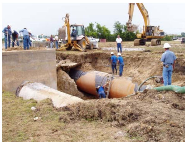
NTMWD personnel make immediate repairs to the failed water transmission pipeline
