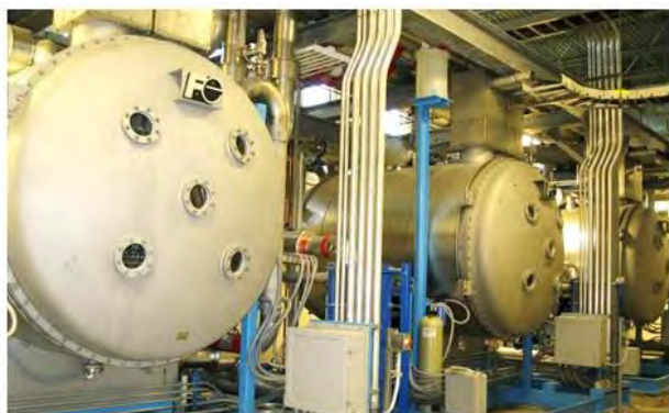
North Texas Municipal Water District Wylie Water Treatment Plant ozone generators. Eleven ozone generators are used to produce up to 3,900 pounds each per day of ozone as the primary disinfectant in the water treatment process.
