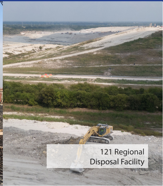
Sister Grove Regional Water Resource Recovery Facility
