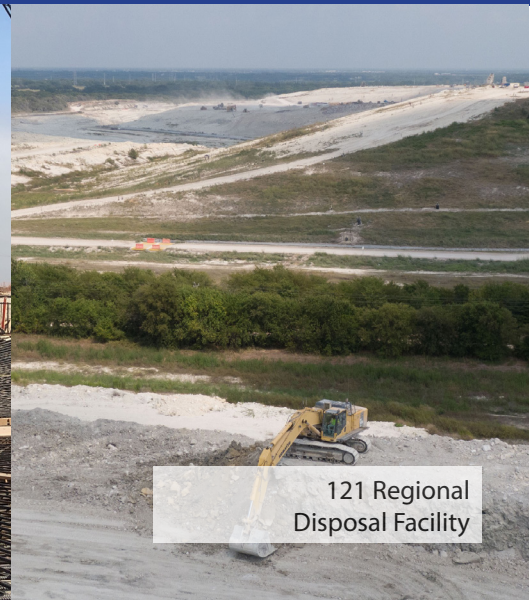
Sister Grove Regional Water Resource Recovery Facility
