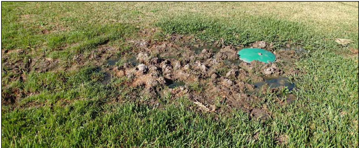
Figure 5.5. Surfacing effluent is a symptom of septic system failure that can be caused by several factors such as poor soil suitability, age of the system, or overloading. Photo courtesy of Texas A&M AgriLife.
