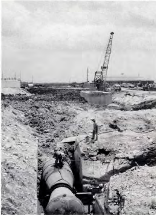
(Left) Apollo Reservoir and Pump Station, the first link to the City of Richardson, can store 5 million gallons of treated water. Built in 1968, the Apollo site also furnished additional delivery and storage for Garland. In the foreground are the 72-inch inside diameter outlet pipeline to the pump station and a 48-inch butterfly valve to control flow. (Right) Apollo to Casa View Pipeline was also part of this new system which helped to provide additional water to Mesquite, Forney, and Kaufman.
