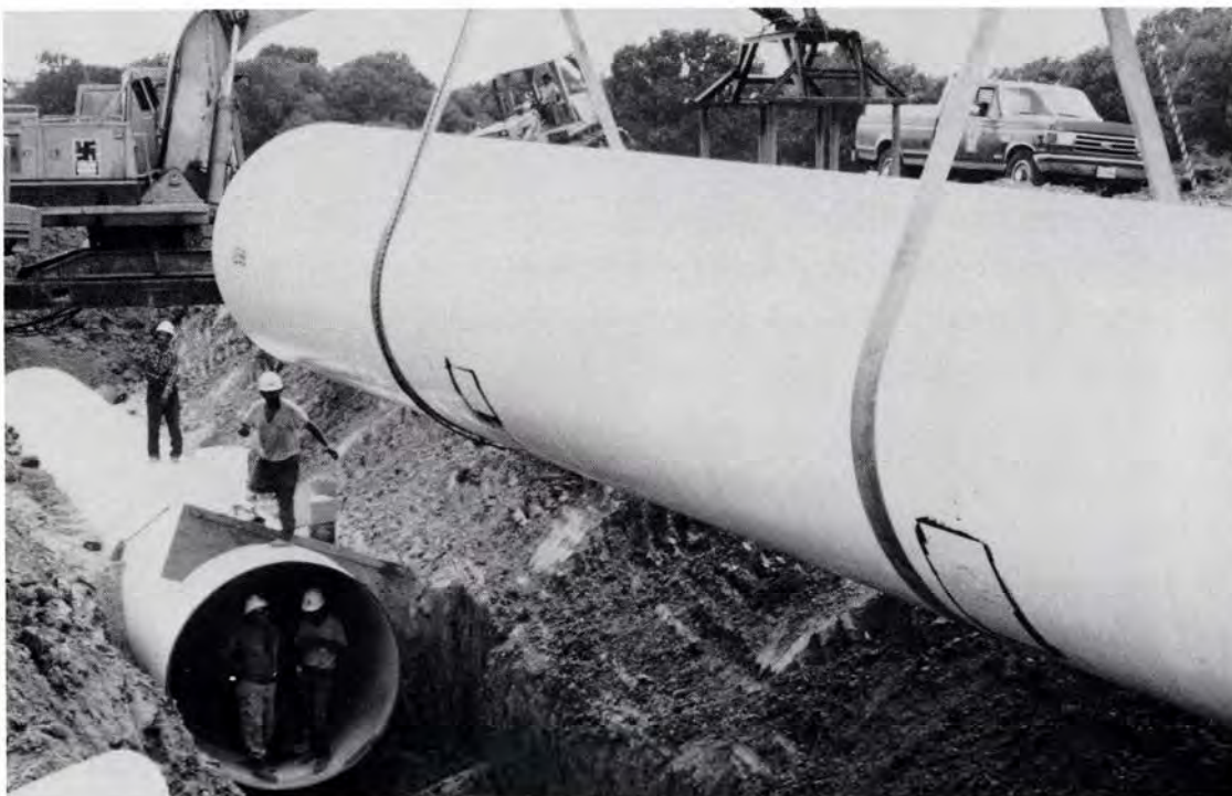
Construction of Cooper Pipeline, Section 2, included 13.8 miles of 84-inch inside diameter pipe installed for the original contract cost of $14,219,523.00.
