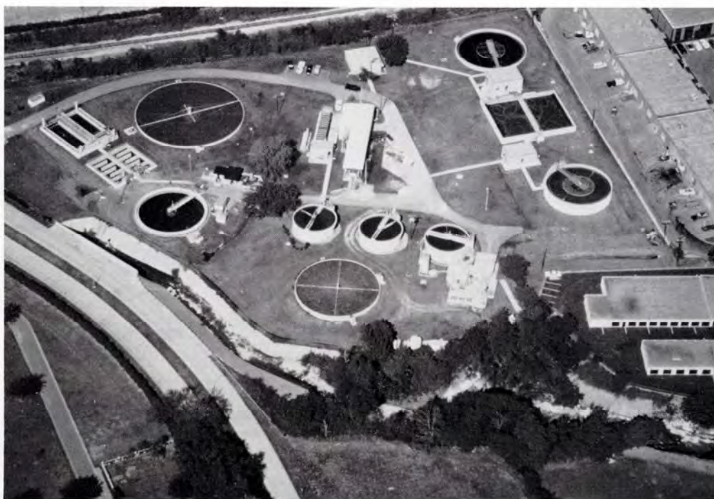
NTMWD Floyd Branch Regional Wastewater Plant, shortly after expansion by NTMWD up to 4.75 MGD from 2.25 MGD. This expansion added a second treatment train, advanced secondary treatment processes, and included filtration and chlorine disinfection.
