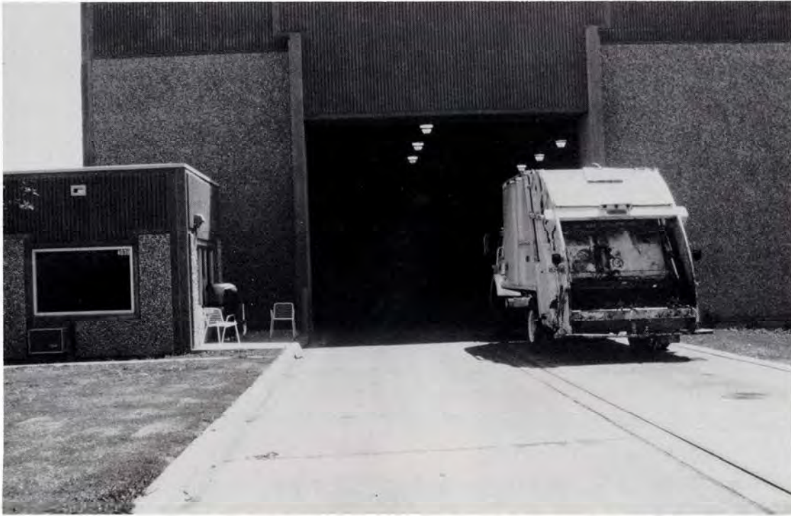
NTMWD Parkway Transfer Station was the first transfer station constructed in the NTMWD Regional Solid Waste System. It opened in 1984 with a capacity to process 750 tons per day through hydraulic push pits in the enclosed building.
