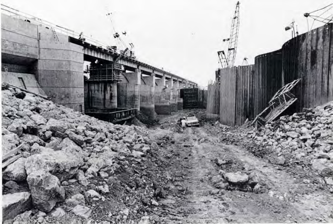
Zachry Co. working on raising the tainter gates on Lavon Dam Enlargement between 1970 and 1973.
