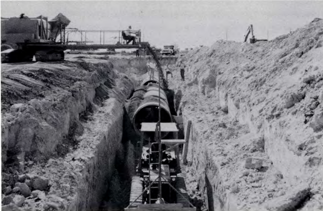
Construction of Texoma Pipeline Section II shows the contractor backfilling around the pipe. Section II included six miles of 72-inch inside diameter pipeline. Total cost for all of the pipeline was over $1 million per mile.
