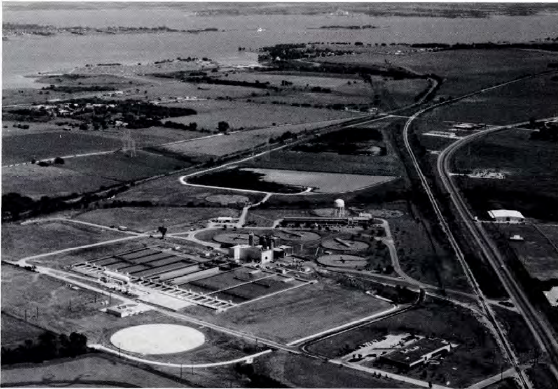
NTMWD Water Treatment Plants I and II in 1987, about the time that a $9.7 million contract was awarded for the final expansion of Plant II. Before the expansion, total treatment capacity was 245 million gallons per day (MGD), while afterwards the plants could treat 350 MGD. In 1958, the original phase of Plant I could treat 20 MGD.
