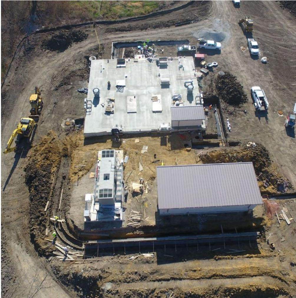
A new lift station in Princeton will soon be online. Construction on the 8 MGD lift station on CR 400 near FM 982 began in September of 2017 with completion scheduled for April. The new \$8.2 million wastewater component will provide additional capacity needed to meet current and future projected peak flows due to population growth in Princeton. Future construction can expand the lift station's capacity to 25 MGD.
