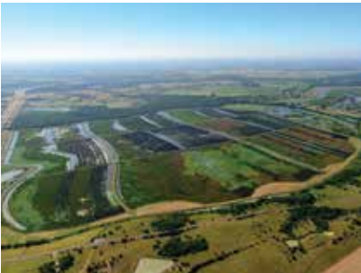
East Fork Water Reuse Project (Wetland)
