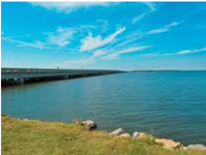
Lake Tawakoni (through a contract with the Sabine River Authority)
