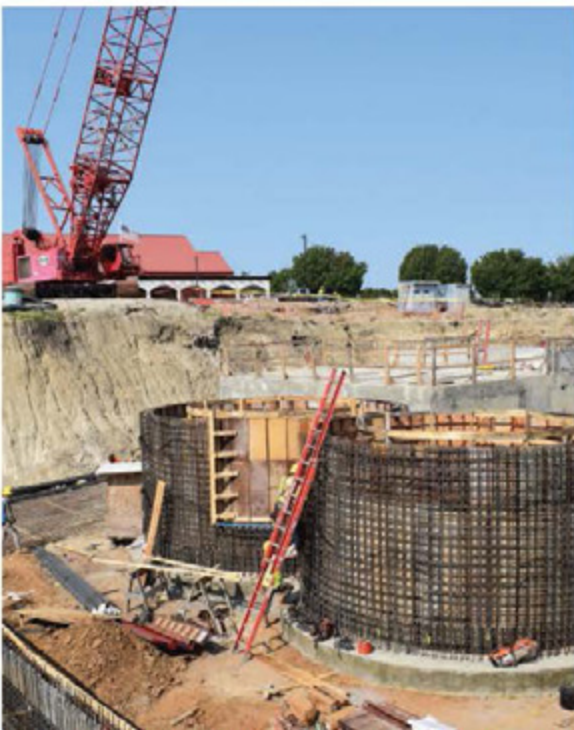
Wilson Creek Regional Wastewater Treatment Plant Expansion
