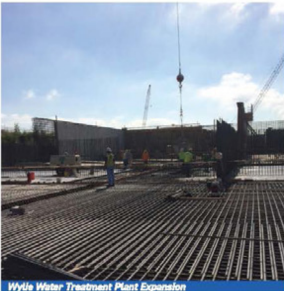
Wylie Water Treatment Plant Expansion
